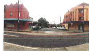
4 EXISTING DEVELOPMENT AT ROSS STREET
